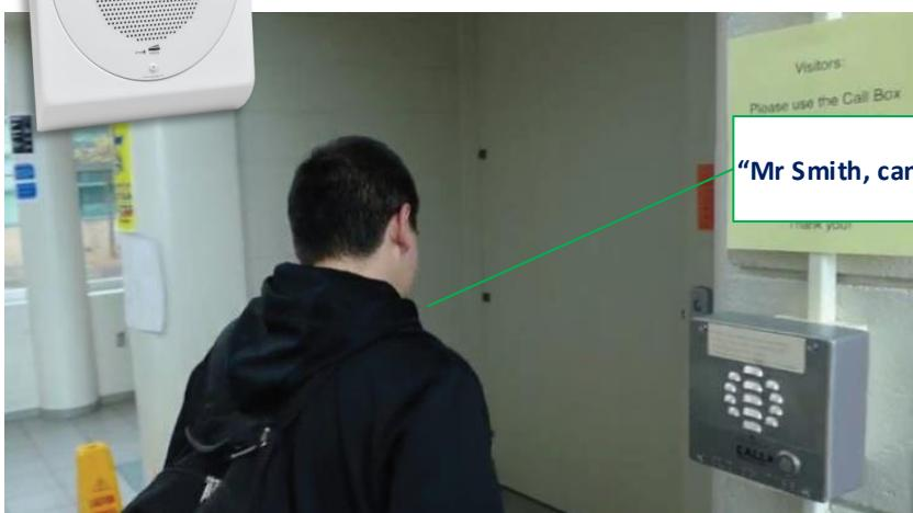
Press the call button on an intercom to call a phone, and a DTMF can be entered to unlock the door.
